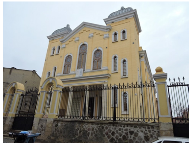
The newly restored synagogue in Edirne
